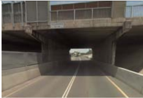
Figure 17.2 Goondoon Street low clearance bridge
