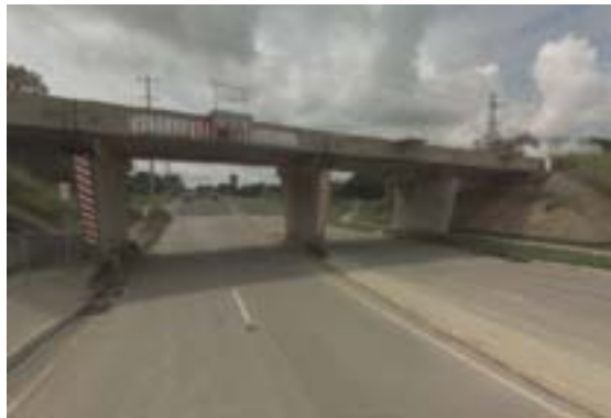
Figure 17.3 Glenlyon Street railway bridge
