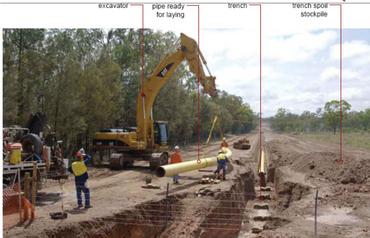
Figure 7.2 Typical pipeline construction – lowering pipes
