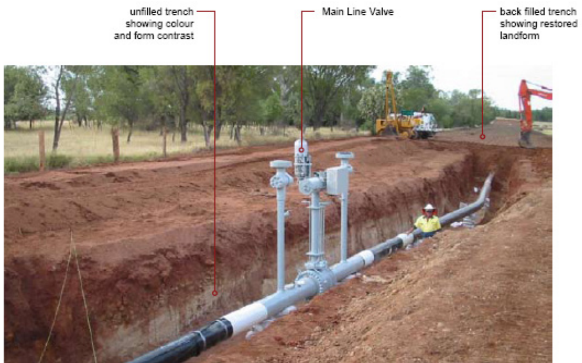
Figure 7.3 Typical pipeline construction – mainline valve
