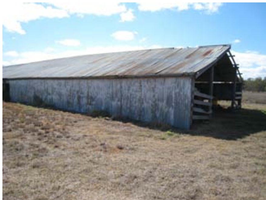
Figure 19.1 Remaining shed used for Cactoblastis breeding at Chinchilla's 'Bug Farm'
